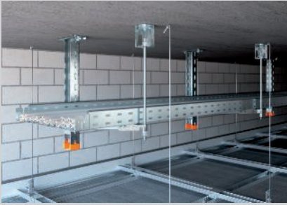
Single-layer ceiling suspension.
