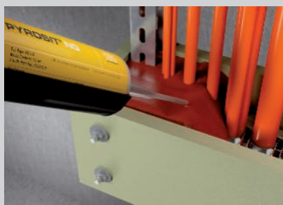
Filling of the cable spandrels with PYROSIT® NG fire protection foam.
