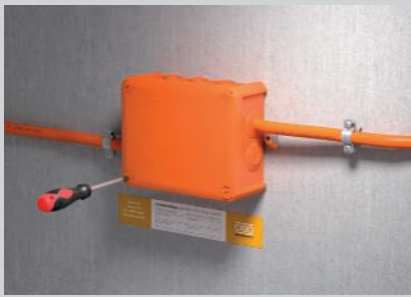
Closing the box with the lid and attaching the identification label.
