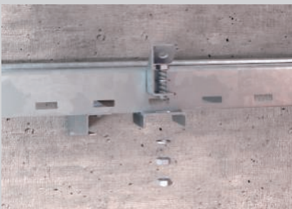
Diagonal mounting of the connection component using hexagonal bolt and hexagonal nuts.
