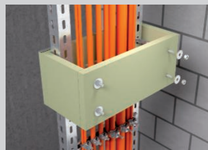
Fastening of the pre-mounted, three-sided housing on the threaded rods.
